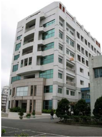
Shore Station north of Taipei, Taiwan
