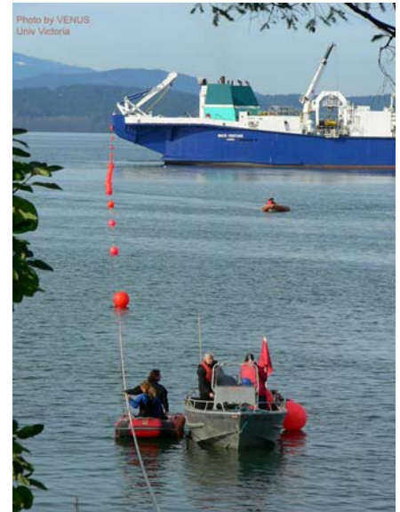
CS Wave Venture Laying Cable
