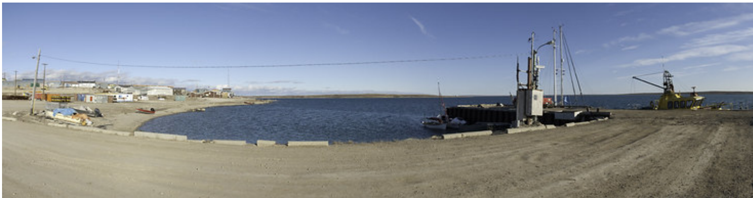
Panorama view of the dock at Cambridge Bay.
