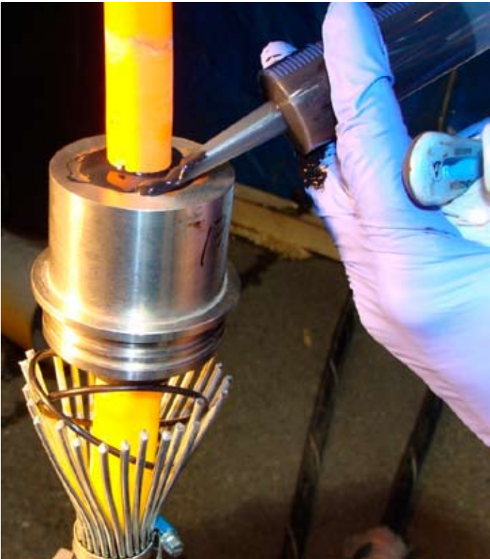
Potting compound applied to the prepared polyurethane jacket. The polyethylene outer jacket is sealed by mechanical means.
